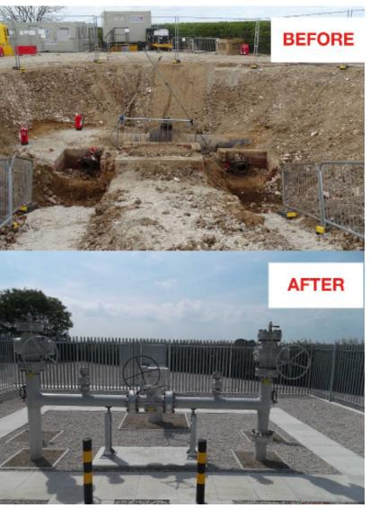
This presented its own difficulties because that excavation had been backfilled with pea shingle, a very loose material which is good to vac-ex but not very stable for heavy plant. Because of this, a change to our temporary works design was required.
