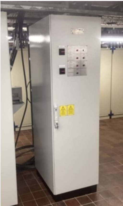
Figure 36: New SIS control panel installed in switch room
