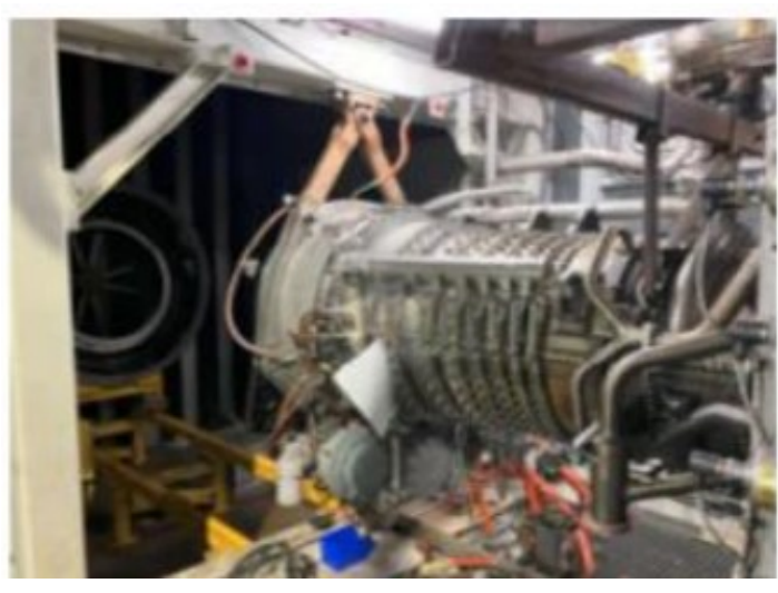
Figure 45: [redacted] Unit 2A - Gas generator removed from container and installation in package in process
