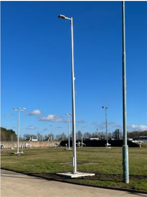
Figure 54 – new road lighting with old still in place (awaiting removal)
