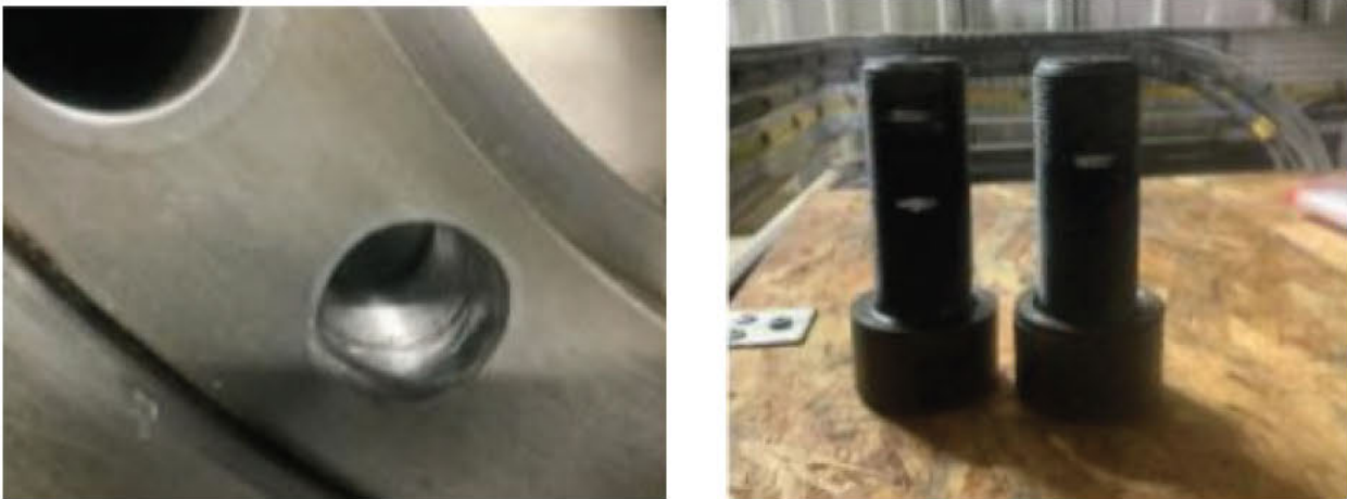
Figure 40: ██████████ Unit 2A -- Bearing flange holes polished and tapped out and bearing assembly bolt showing new thread
