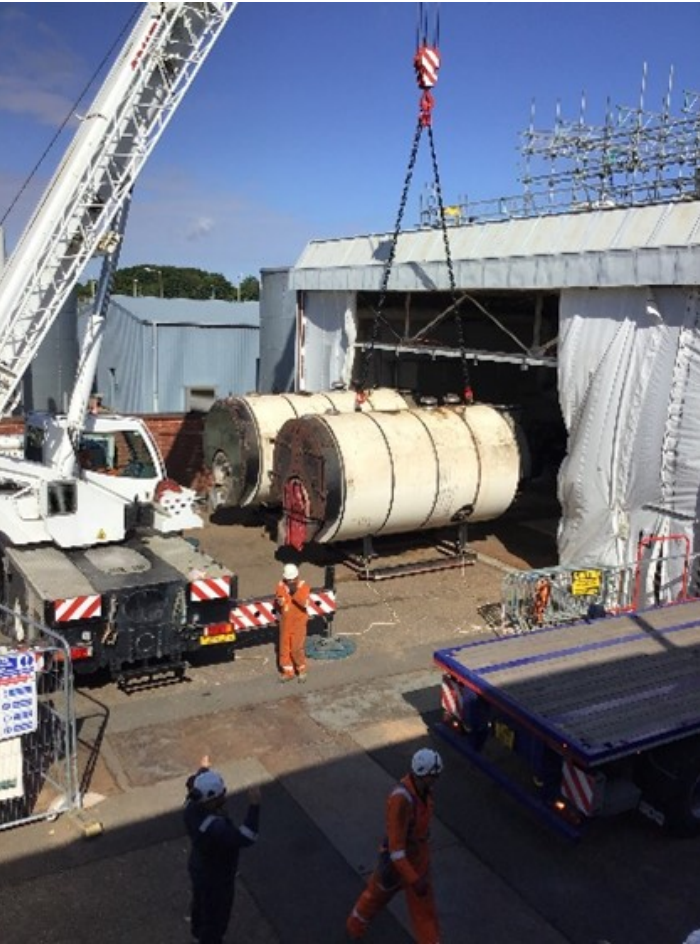
Figure 58: Boilers being removed from boiler house 2.
