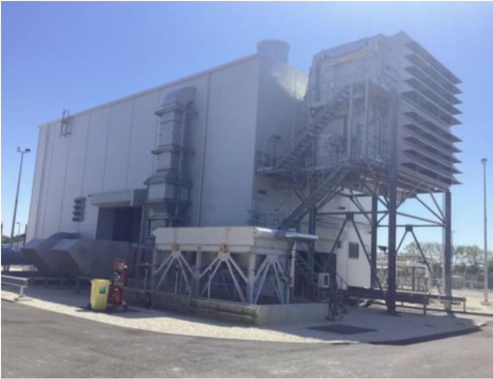
Figure 25: Completed cladding and air-intake HVAC works
