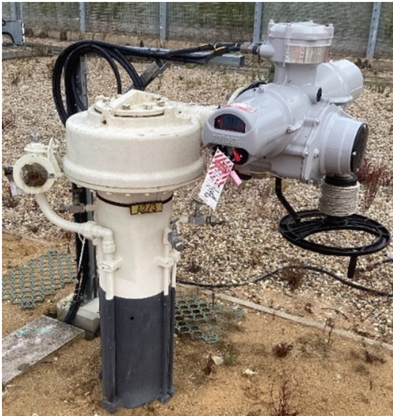
Figure 35: Perenco 2 new Rotork actuators installed for closure of A2/3 valve as part of SIS
