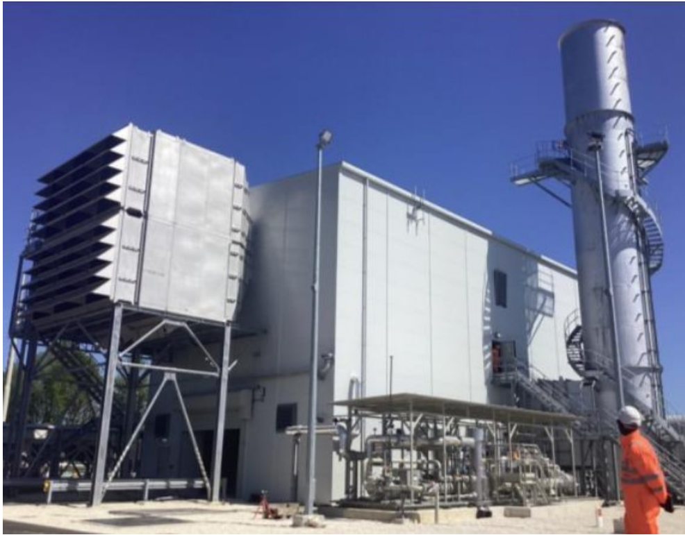
Figure 27: Completed fuel gas skid and exhaust stack
