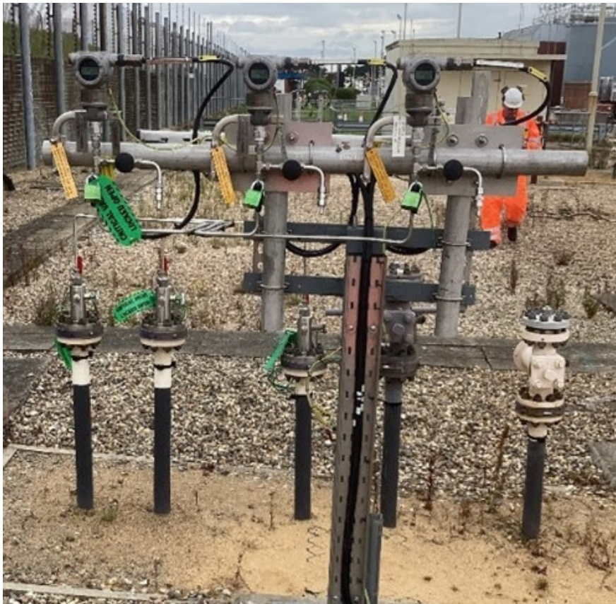
Figure 34: Perenco 1 pressure transmitters for the safety instrument system (SIS) voting system for final elements
