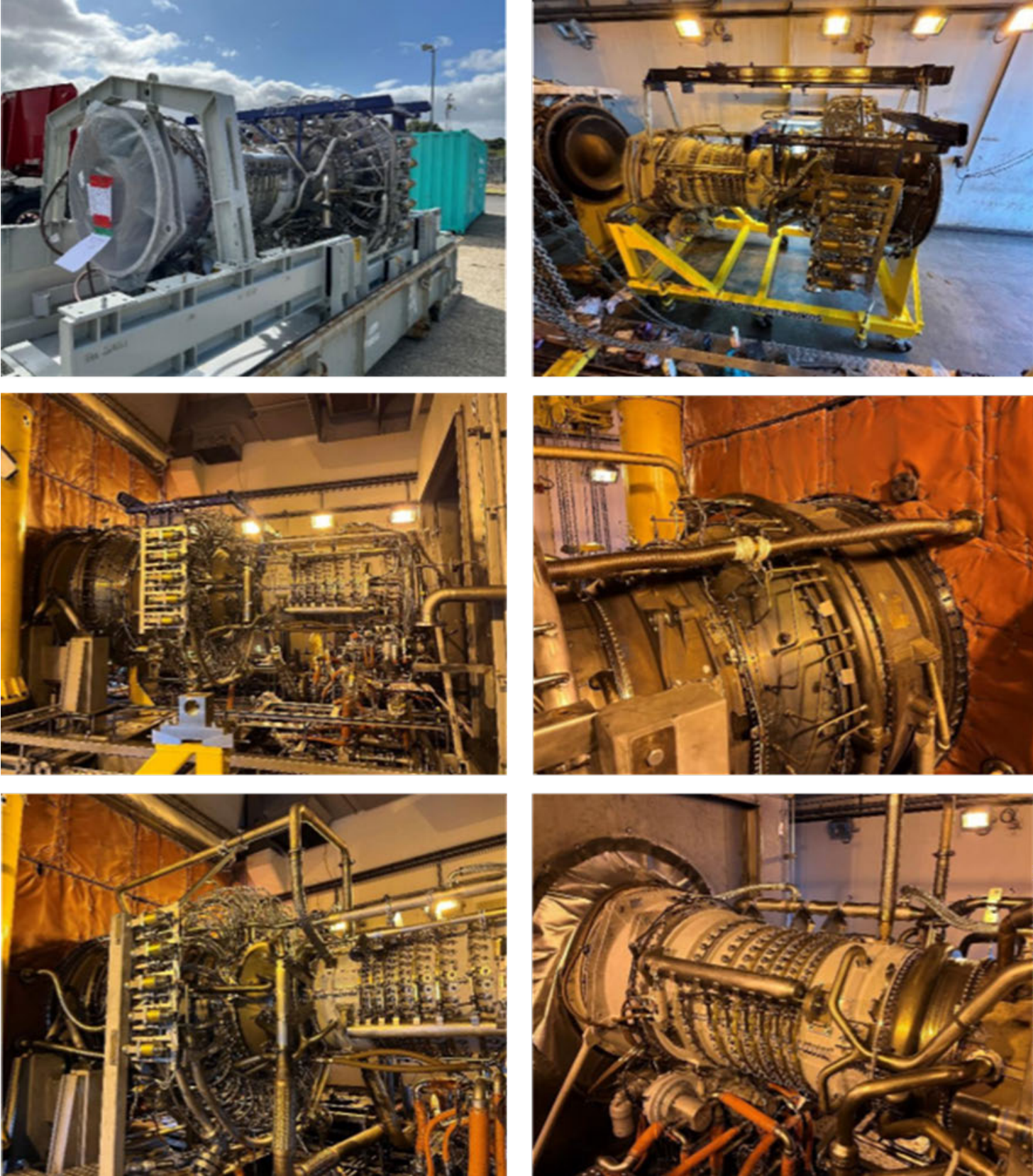
Figure 46: [REDACTED] Unit A - Installation of gas generator - new engine hoisted into package before being installed
