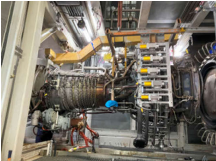
Figure 44: [redacted] Unit 2A - Removal of gas generator
