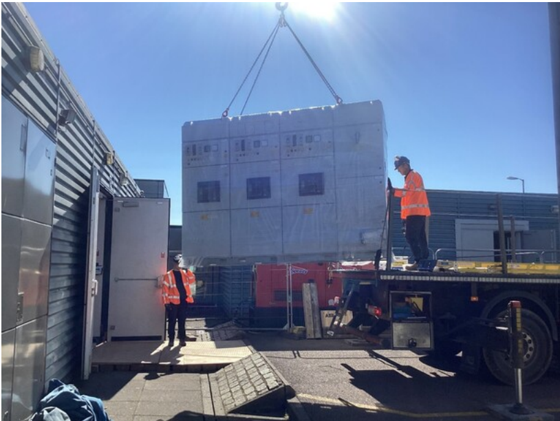
Figure 55– [REDACTED] Voltage switchboard (Air Circuit Breaker section) being delivered to site
