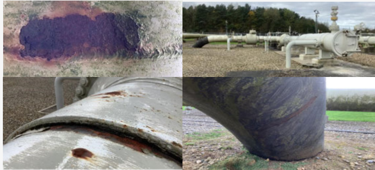
Image 7 – 10: Site Condition prior to intervention [REDACTED]
