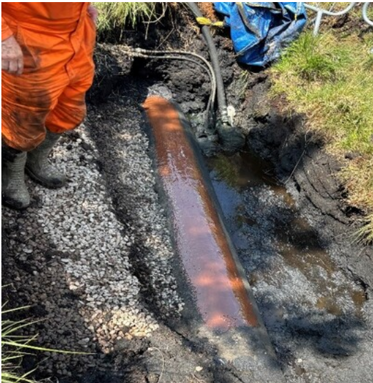
Image 35: Pipeline coating repair and upgrade
