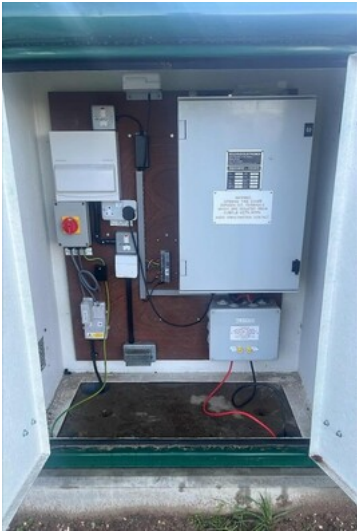
Image 37: Replacement of Transformer Rectifier (TR) and installation of remote monitoring unit (Completed works)
