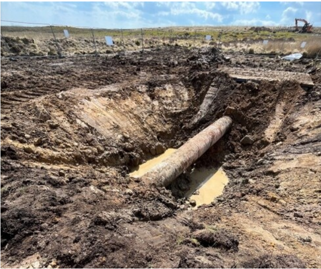
Image 34: Pipeline excavation for coating repair
