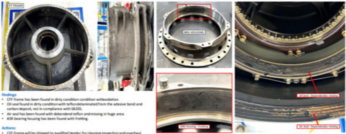
Image 25: [redacted] LM2500 Gas Generator Overhaul – Detailed inspection of the compressor front frame and casing components, identifying wear, surface degradation and areas requiring refurbishment prior to reassembly
