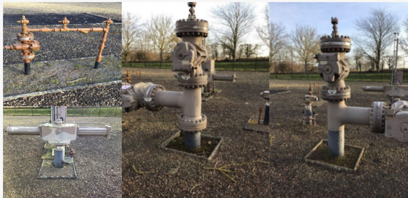
Image 15 – 18: Site condition prior to intervention [REDACTED]
