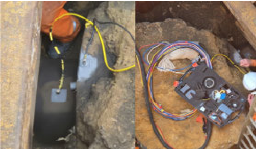
Image 36: Road crossing inspection & test post installation
