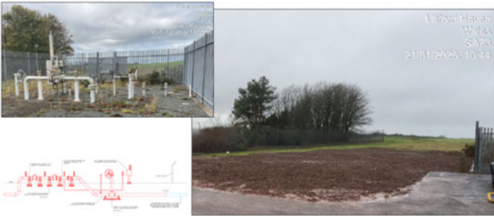
Image 2: Upper Neeson AGI Pipeworks Removal
