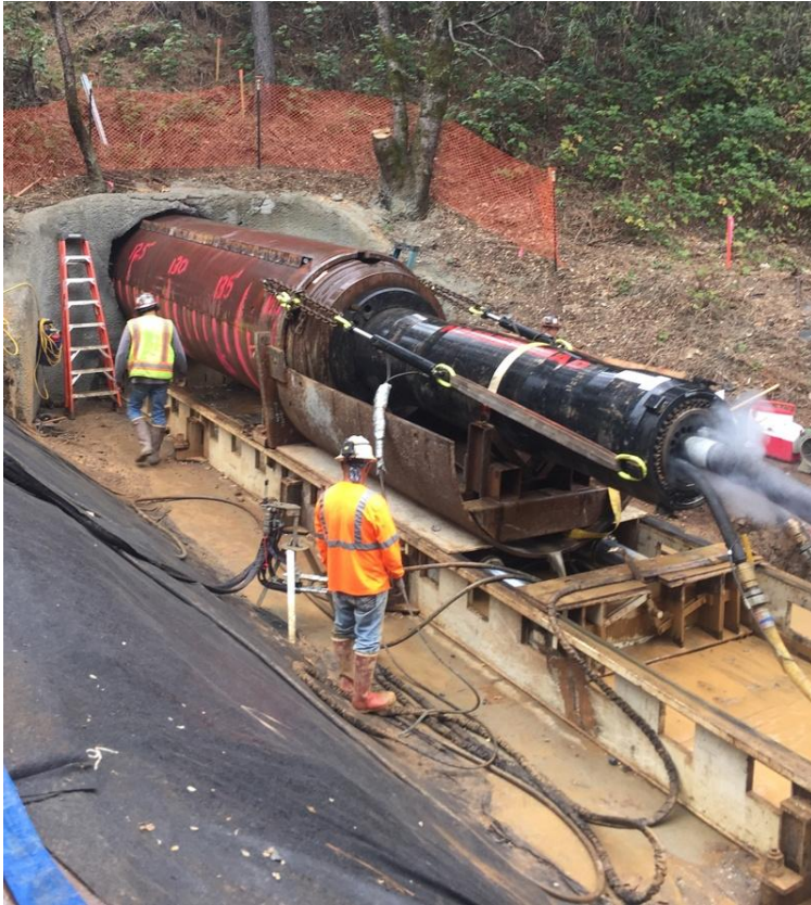
Figure 10 Pipe Ramming (Image from www.ukstt.org.uk )
