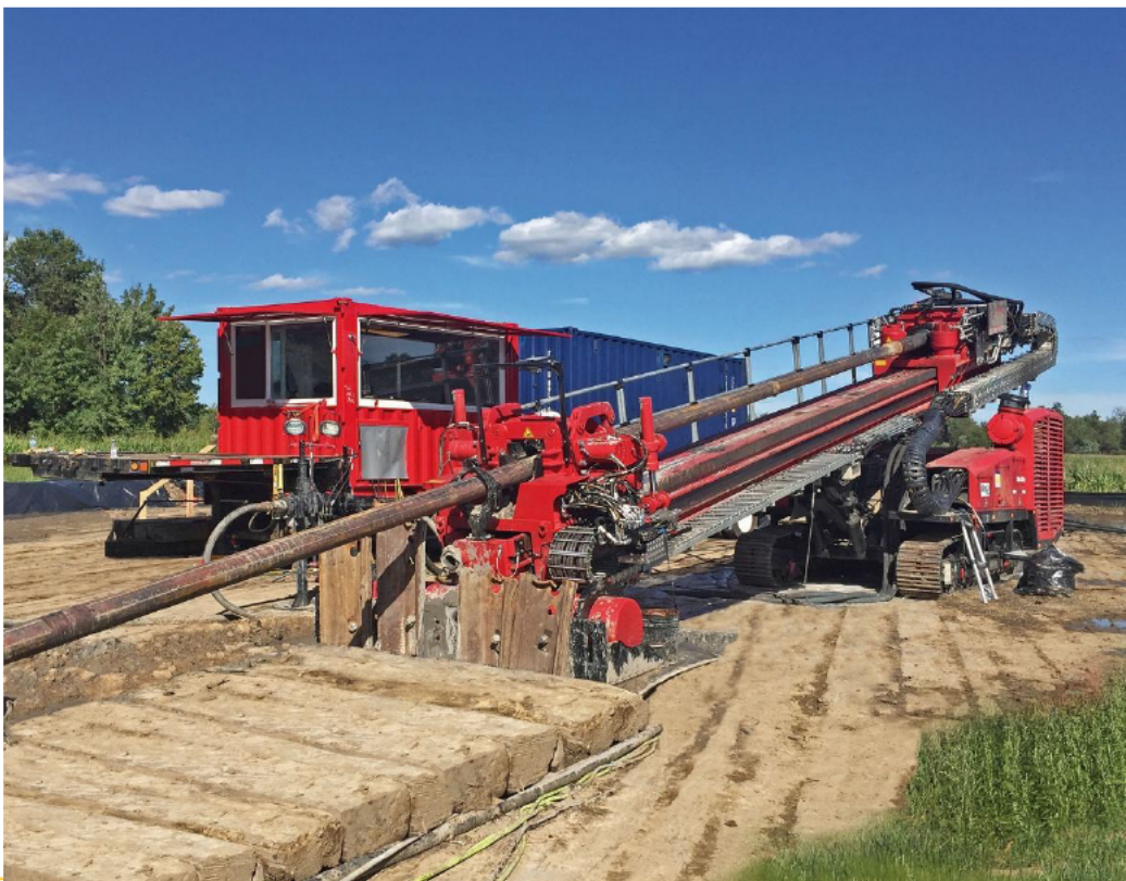
Figure 6 HDD Rig (Image from prime-drilling.de )
