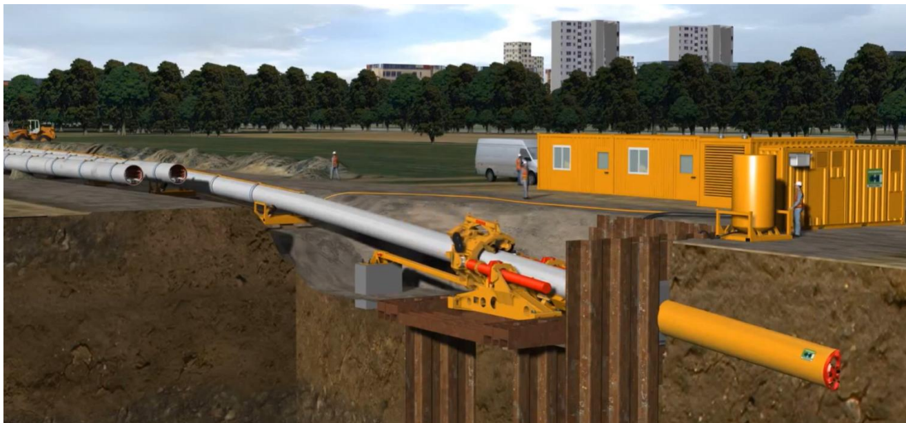
Figure 11 Direct Pipe® (Image from www.herrenknecht.com )
