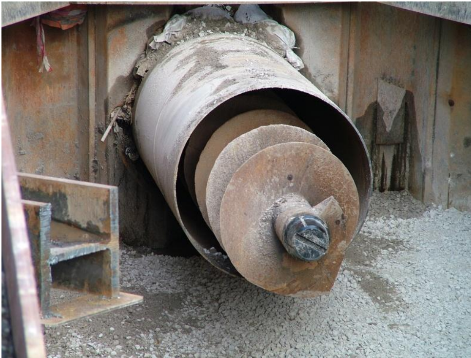
Figure 9 Auger Boring (Image from www.ukstt.org.uk )
