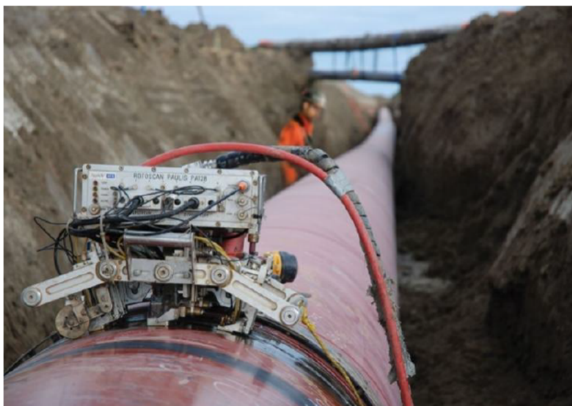
Figure 20 Applus Rotoscan Automated Ultrasonic Inspection
