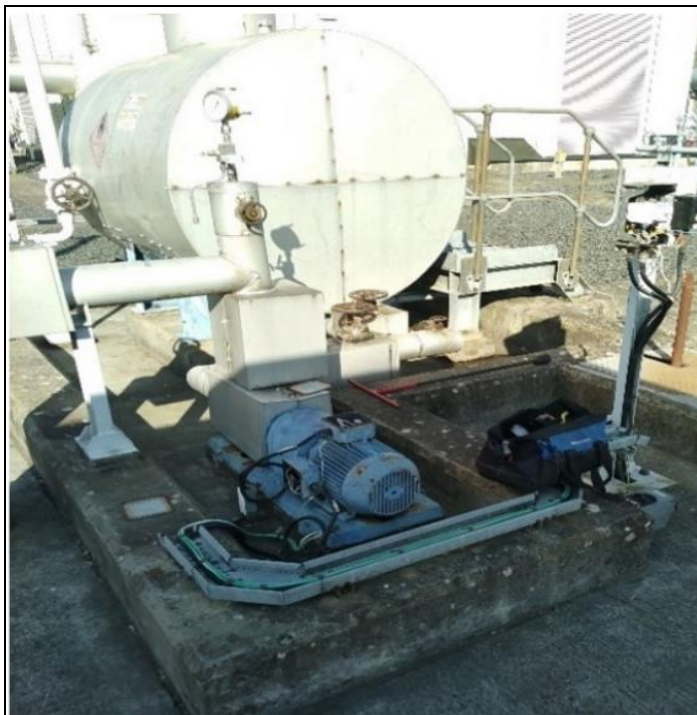
Figure 7: Lubrication System
