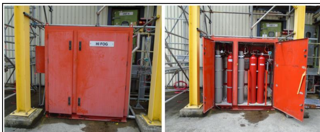
Figure 9: Water Mist Kiosk and Cylinders
