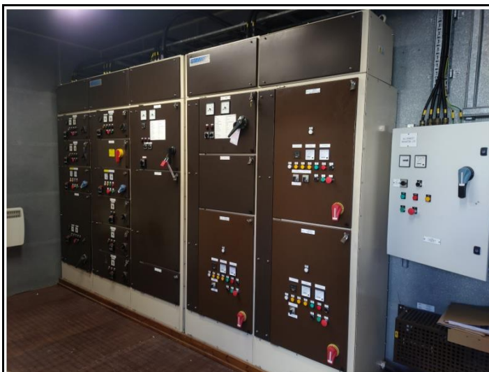
Figure 11: AC MCC (Left) and DC MCC (Right)
