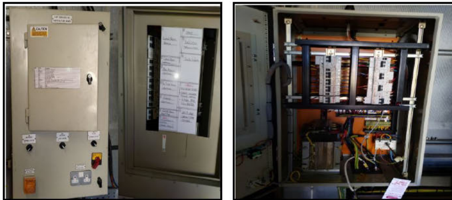
Figure 12: AC Unit Services DB External (Left) and Internal view (Right)
