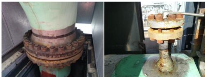
Figure 18: Coating breakdown on Acoustic Enclosure Flange
