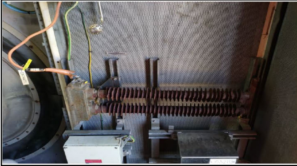
Figure 13: Gas Turbine and Compressor Area Heaters (typical of all)
