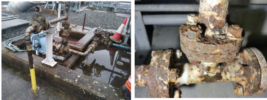
Figure 17: General condition of lube oil pipework (left) and Flanges (right)
