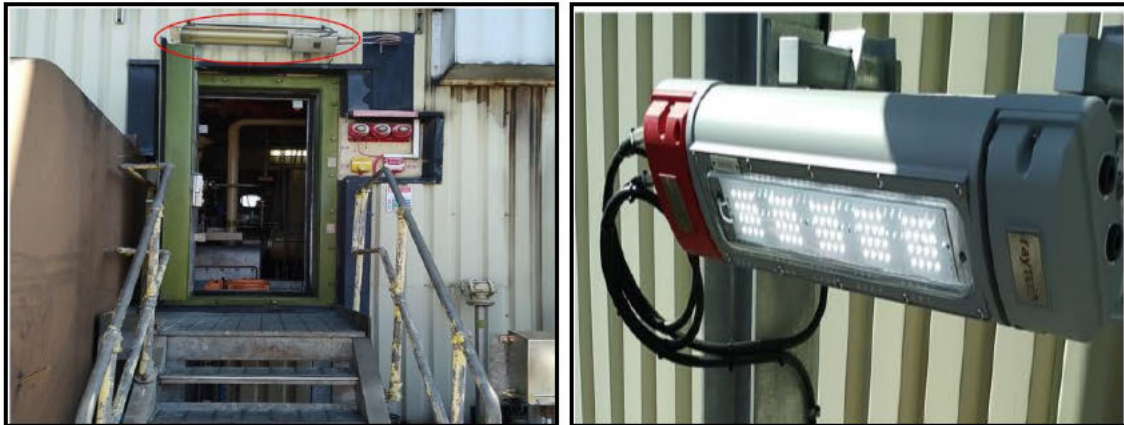
Figure 14: Fluorescent CAB lighting (left) and LED stairway lighting (right)
