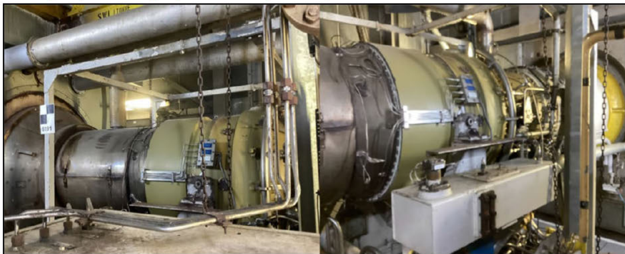
Figure 3: St. Fergus Unit 1A Gas Generator
