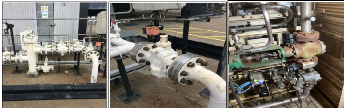
Figure 23: Unit 1A Fuel Gas arrangement
