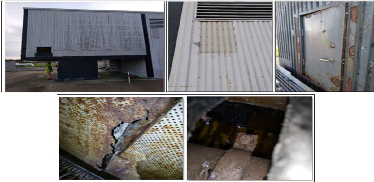
Figure 26: Unit 1A Outer CAB: Pictures depicting hole in the lined panel and submerged baseplate
