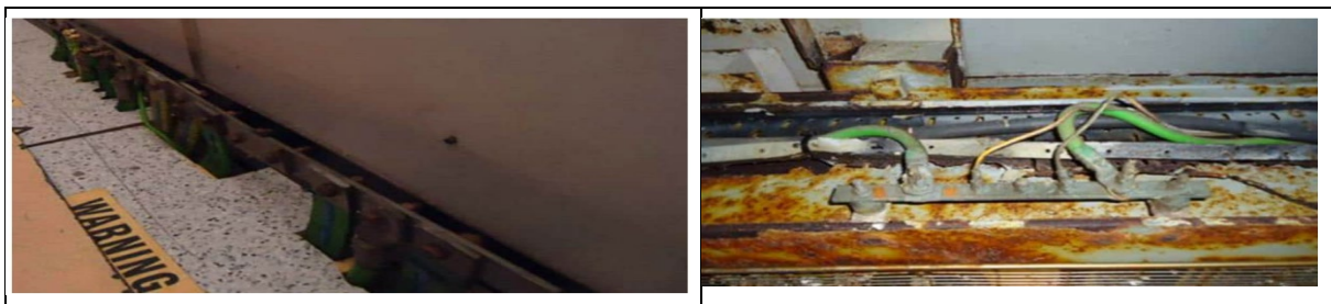
Figure 35: Condition of typical earthing supporting Unit 1A
