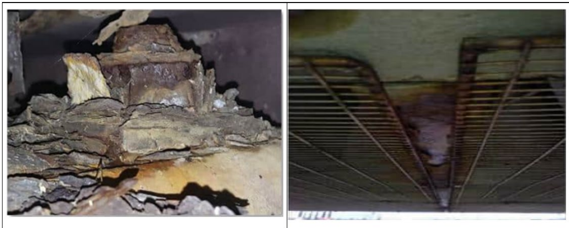
Figure 25: Unit 1A Air Intake: Pictures depicting corroded FOD mesh and baseplate fixing
