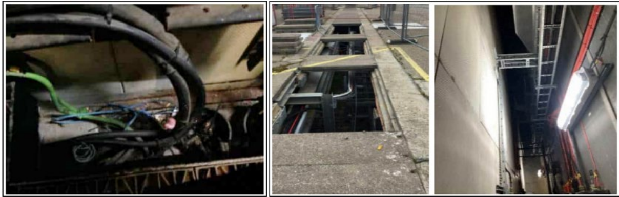
Figure 15: Representative cable runs and trays supporting Unit 1A
