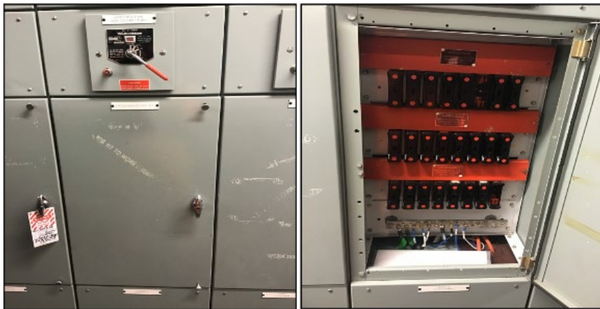
Figure 33: Unit 1A Individual distribution board within J1(Interior and exterior)
