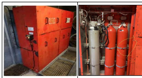
Figure 28 29: Unit 1A Fire suppression system cabinet (Interior and exterior)
