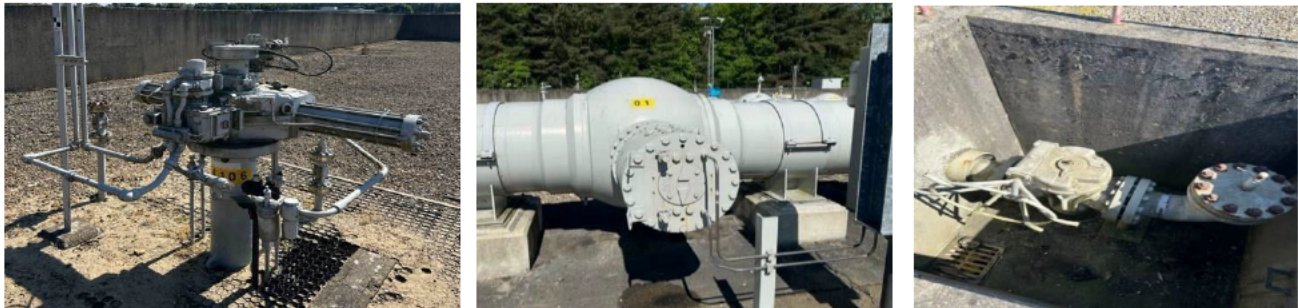
Figure 1: Below ground valve and its above ground operator, above ground valve and a valve in a pit.
