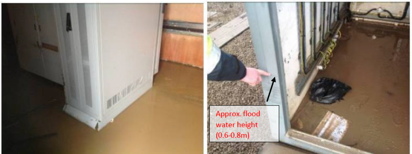
Figure 11: Internal and External Flood Damage, Flood-water Height in Most Places was between 0.6 to 0.8m
