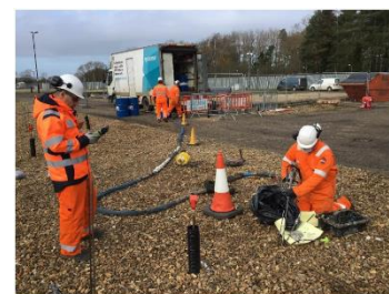
Figure 12 – Injection & Live Monitoring
