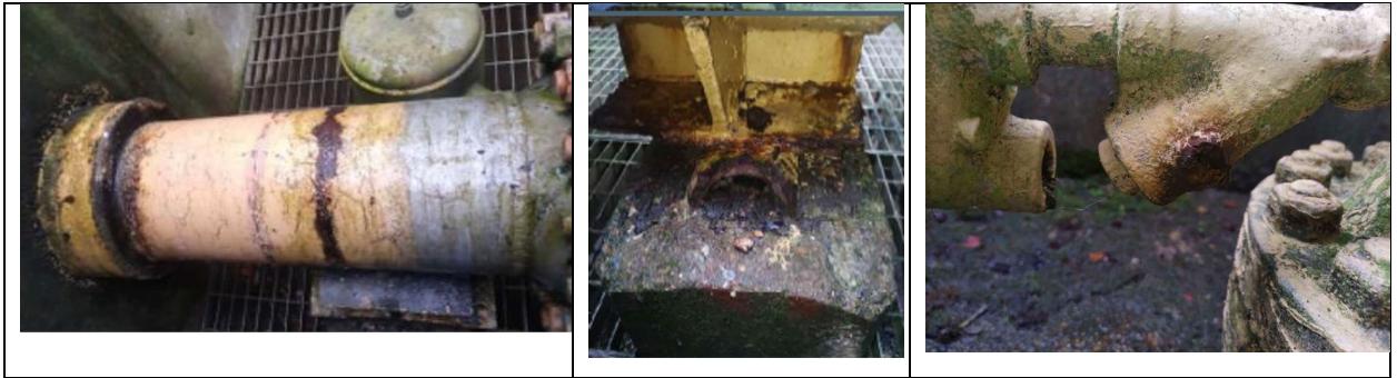
Figure 4: Pipework corrosion and damage
