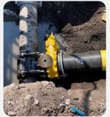
All network documentation and supervision required for the new gas connection to the 8-inch steel parent main was carried out following detailed site specifications for the installation along with testing of the outlet pipework to conform with the internal permit requirements to allow the adoption of the works.
