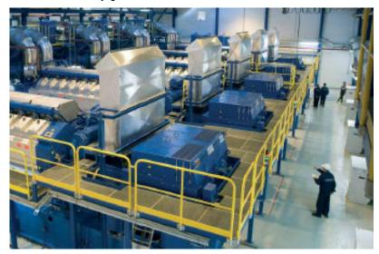
Figure 1: Inside of a gas engine power plant (Wärtsilä)
