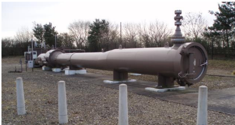
Figure 3.3: An NTS pig trap
