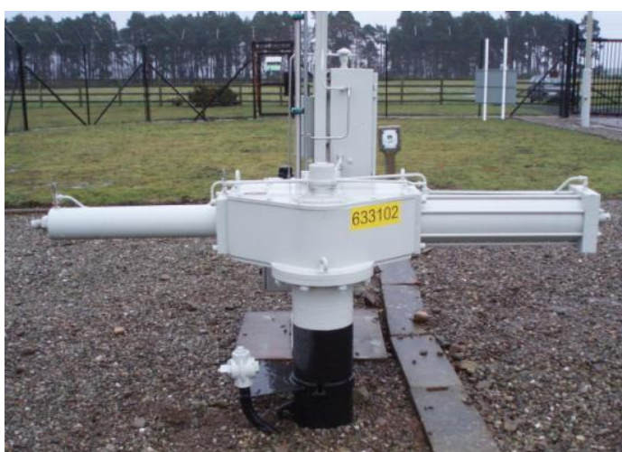
Figure 3.4: A gas actuator on a buried valve
