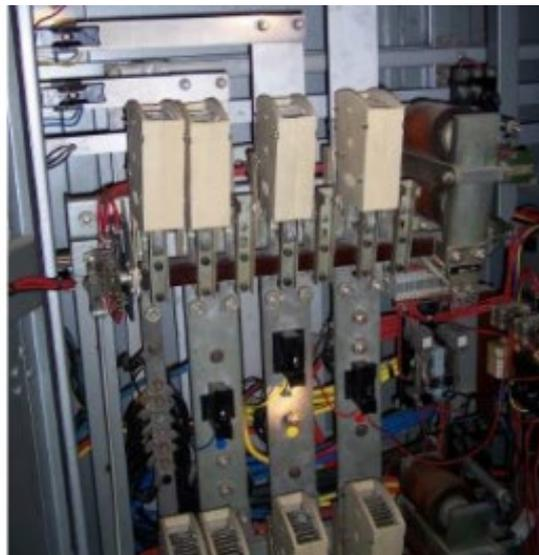
8.4.24 Redundant and oversized circuitry due to changed requirements Over the years, some equipment has had to be disconnected from the LV electrical system due to changes in requirements and regulations. This has led to redundancy of some circuitry and distribution boards.
