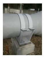
To date we have installed one composite pipe support at Bishop Auckland Compressor Station through our National AGI Renovation Campaign (NARC). We are monitoring this to ensure its' fitness for purpose in the field.
