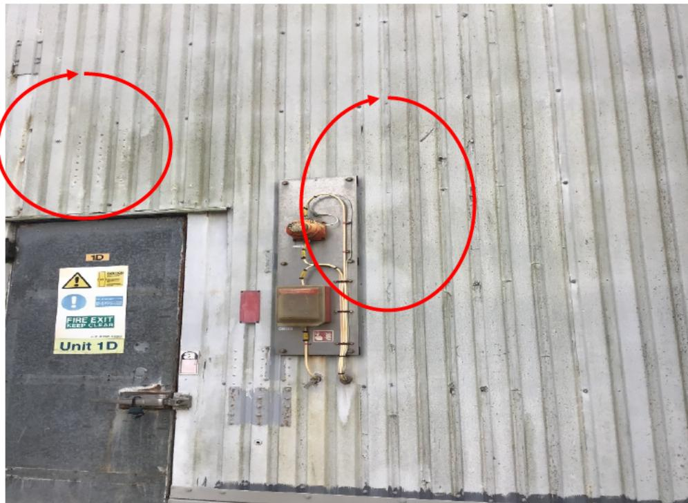
Figure 8: Flaking Cladding on 1D
