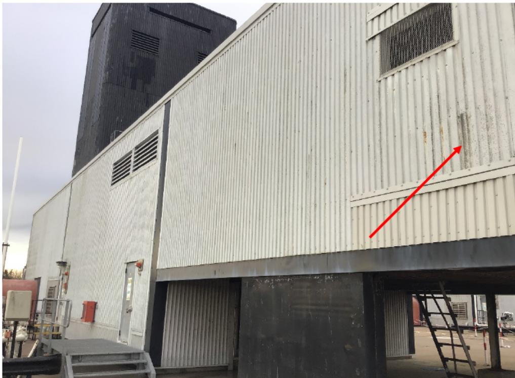
**Figure 6: Flaking Cladding on 1A**
