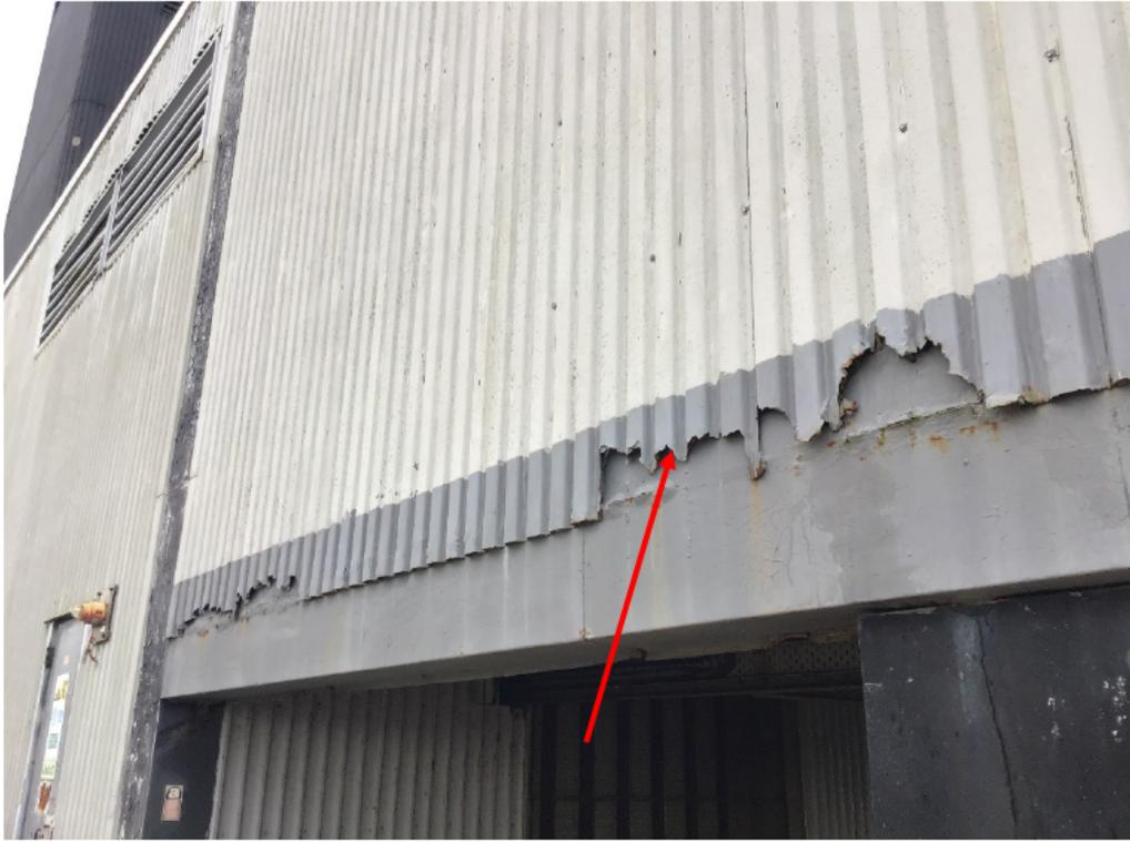
**Figure 5: Flaking Cladding on 1C**
