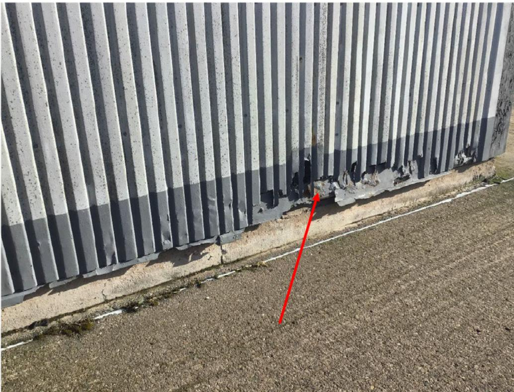
**Figure 4: Damage on 1C Bottom Cladding**
