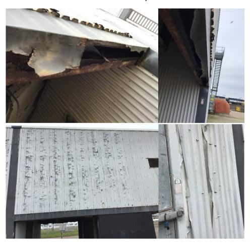
Figure 4: Coating breakdown of Galbestos cladding
