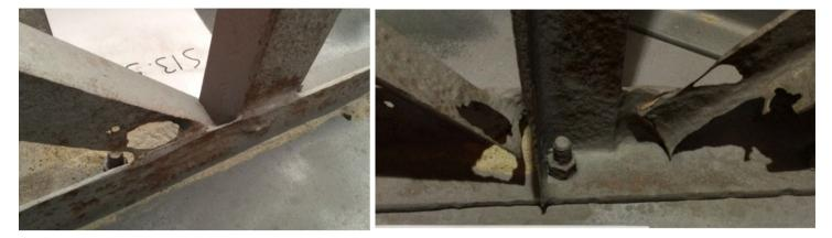
Figure 22 Secondary Lattice Girder Corrosion
