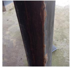
Figure 31 Plant 2 Column 20 Moderate corrosion of column
