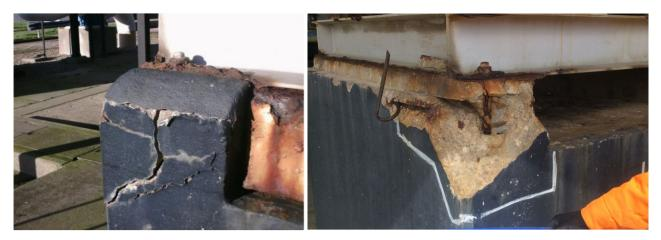
Figure 27 Plant 2 Aftercooler Concrete Fan Plinth cracking Figure 28 Plant 2 Aftercooler Concrete Fan Plinth 36 Severe Concrete Issues
