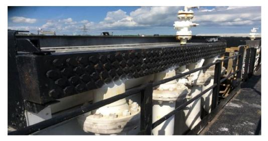
Figure 11 Tube Plugs on Header Box
