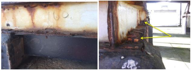
Figure 29 Photos Highlighting Corroded Fan Main Anchor Bolts
