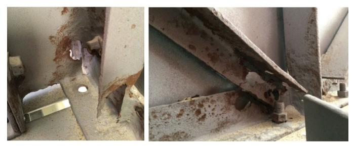
Figure 20 Aftercooler Frame Corrosion
