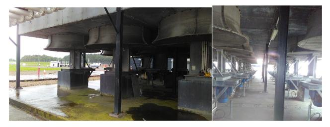
Figure 24 Sections of Concrete Foundation and Fan Plinths at Plant 1 Aftercooler
