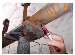
Figure 10: Through wall corrosion leading to pinhole leak requiring replacement
