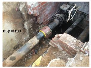
Figure 12: Temporary Plidco Clamp on Actuating pipework at pit wall transition
