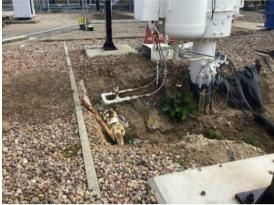
Figure 44: Corrosion and ground movement threats to Actuators
