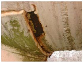
*Figure 6: Actuating pipe clashing with main gas line due to ground movement*
