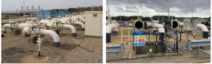
Figure 22: Class 600 Horizontal Filter Vessel
