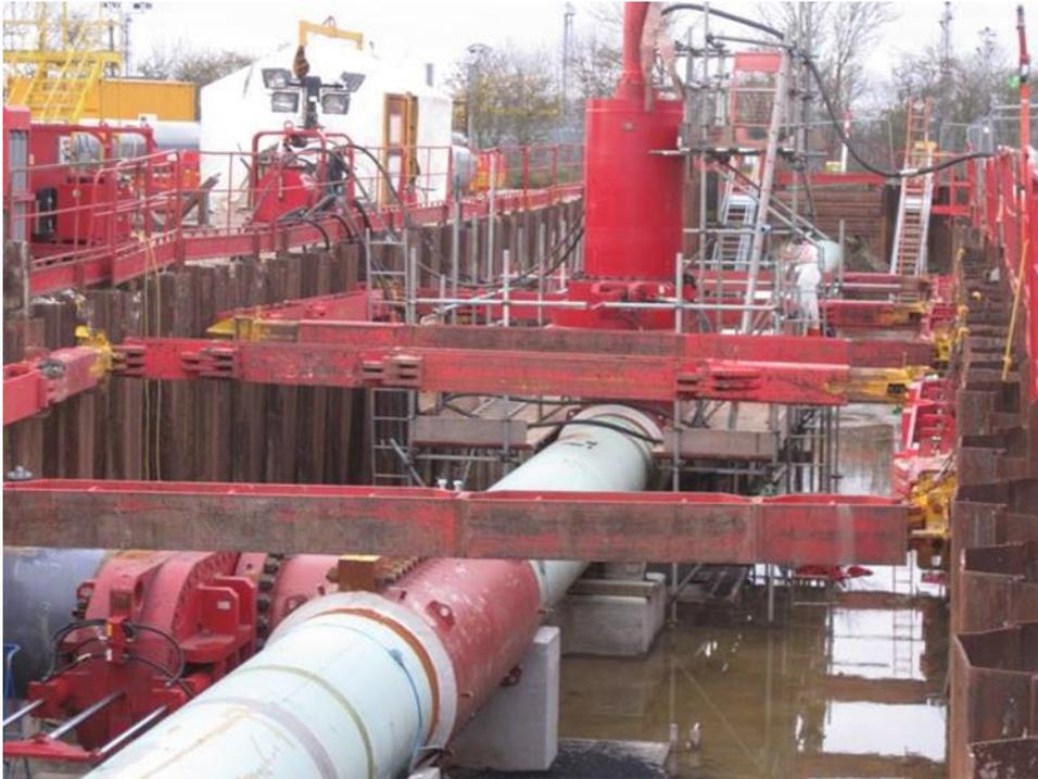
**Figure 22: Temporary By-pass pipeline installation and drilling tool in situ – Goxhill**
