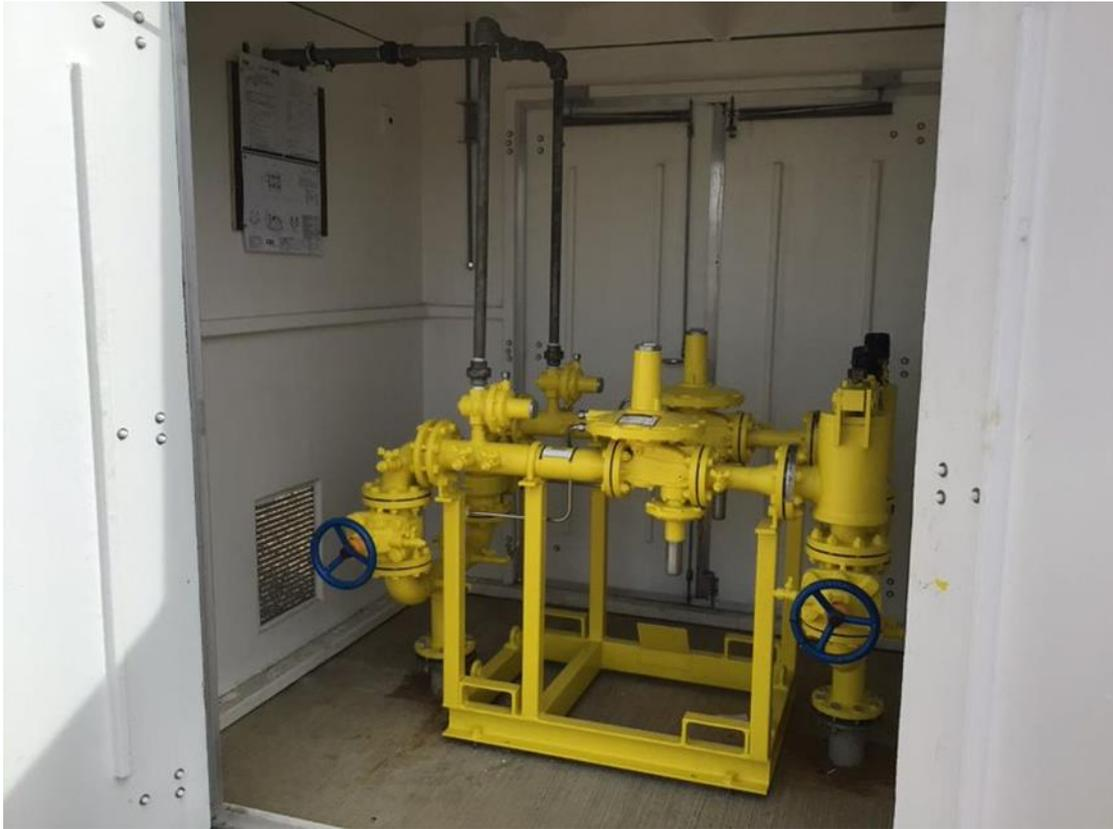
**Figure 9: Simplified pressure regulator installation for boiler fuel gas**
