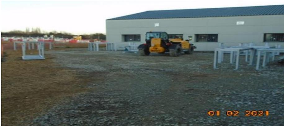
**Figure 25: Telehandler moving Panel supports into the control building at Peterborough**
