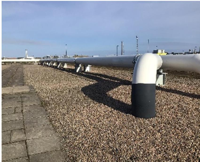
**Figure 12: Freshly painted Ancala pipework and new pipe supports**
