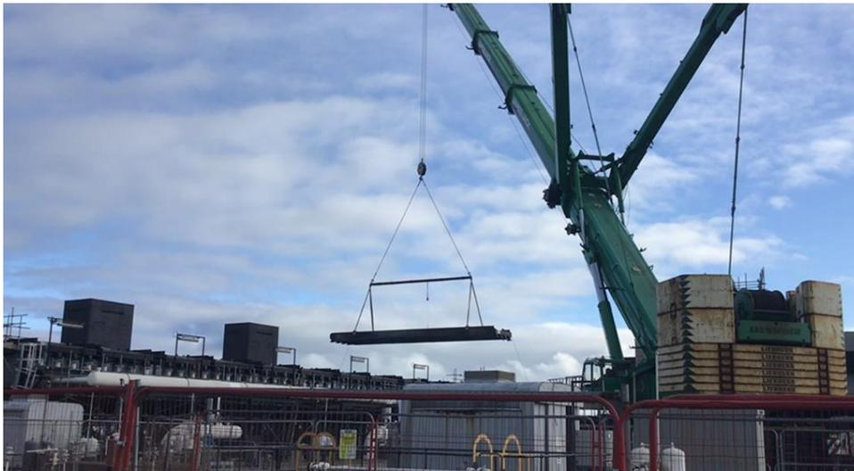
**Figure 13: Old Aftercooler section during removal Autumn 2020**
