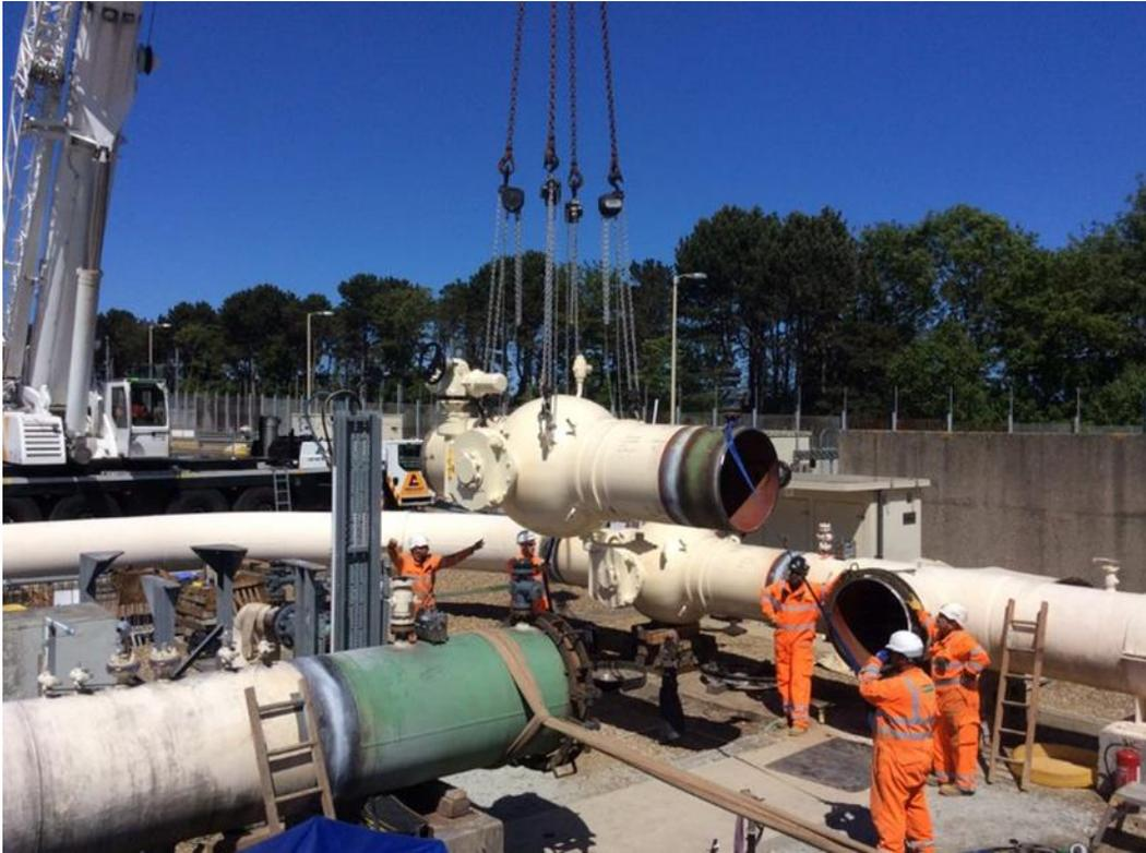
**Figure 7: Valve installation during ‘Phase 8’ works**
