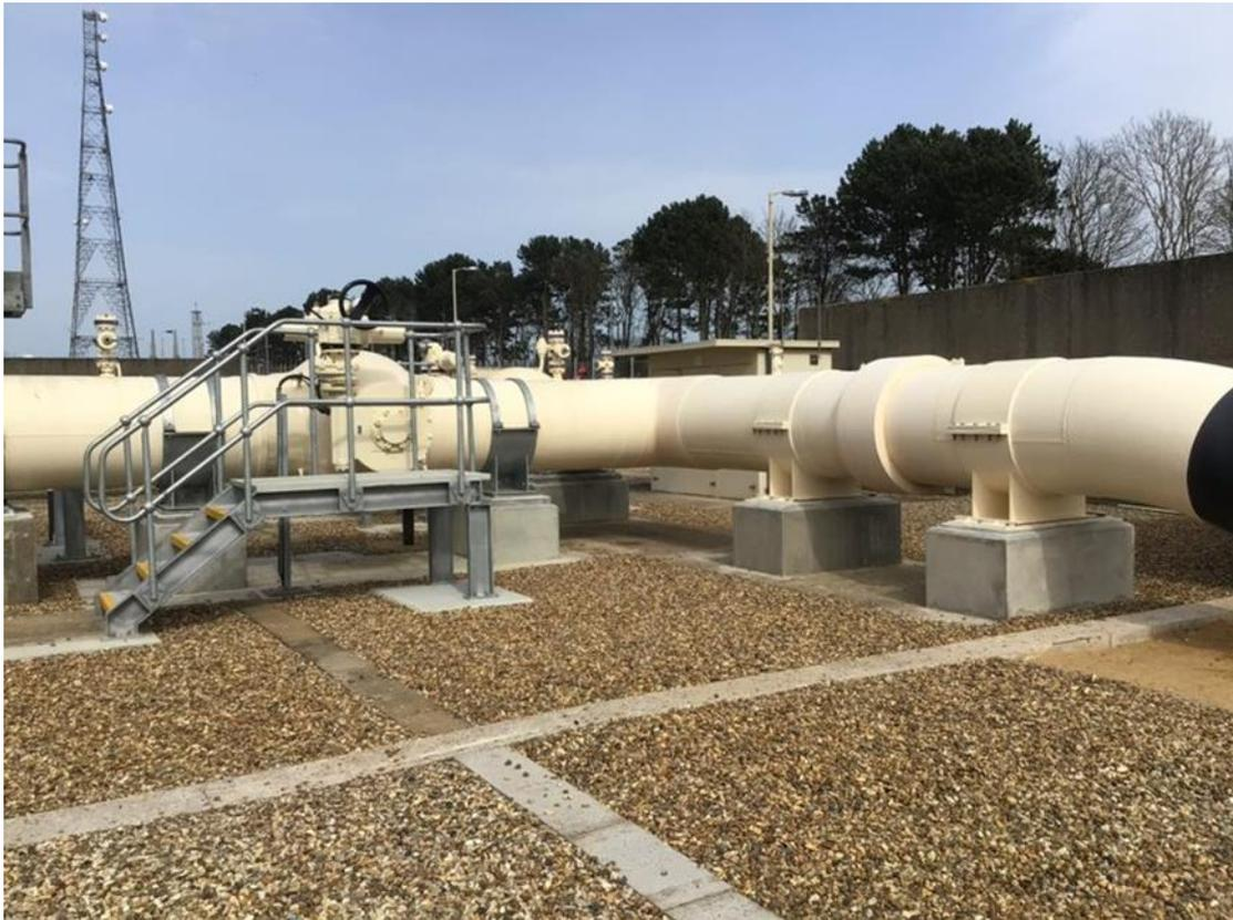
**Figure 8: Final installation paint standard and pipe supports 'Phase 8'**
