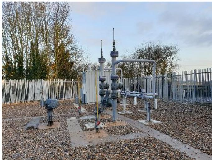
**Figure 4: New and first Biomethane connection to the NTS at Murrow offtake**
