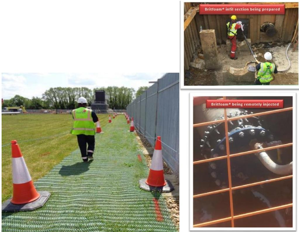
**Figure 19: Eco-walkway at Kings Lynn CS and of the Britfoam being injected**
