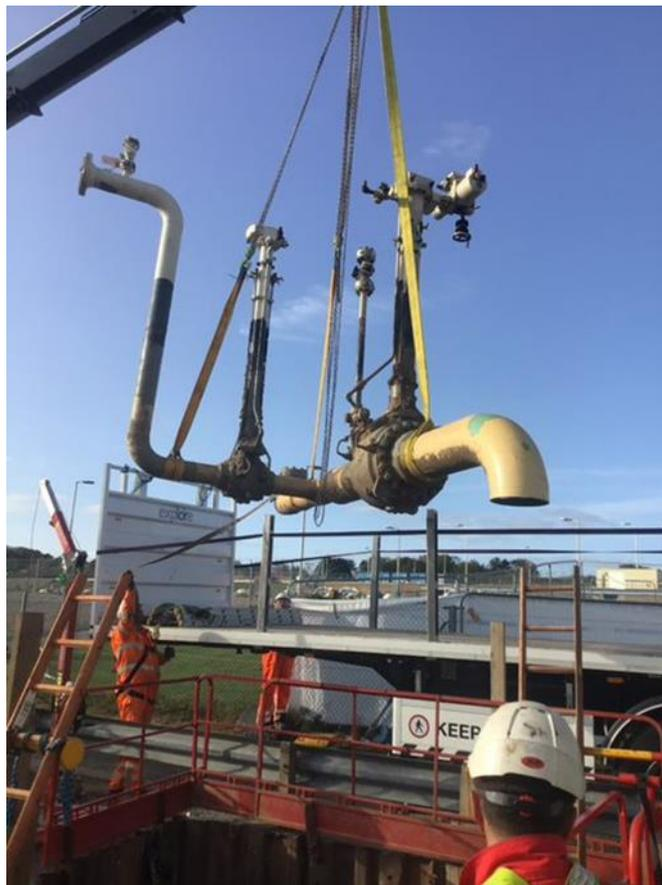
**Figure 6: Removal of old A3/1 valve 'Phase 9'**
