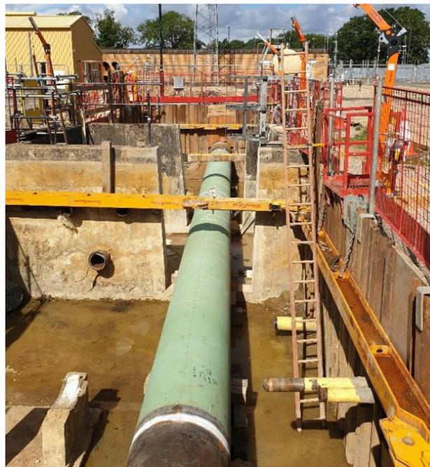
**Figure 18: Network welded into position.**
