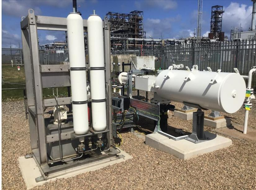
**Figure 11: Electro Hydraulic actuator and associated Hydraulic Power Unit**
