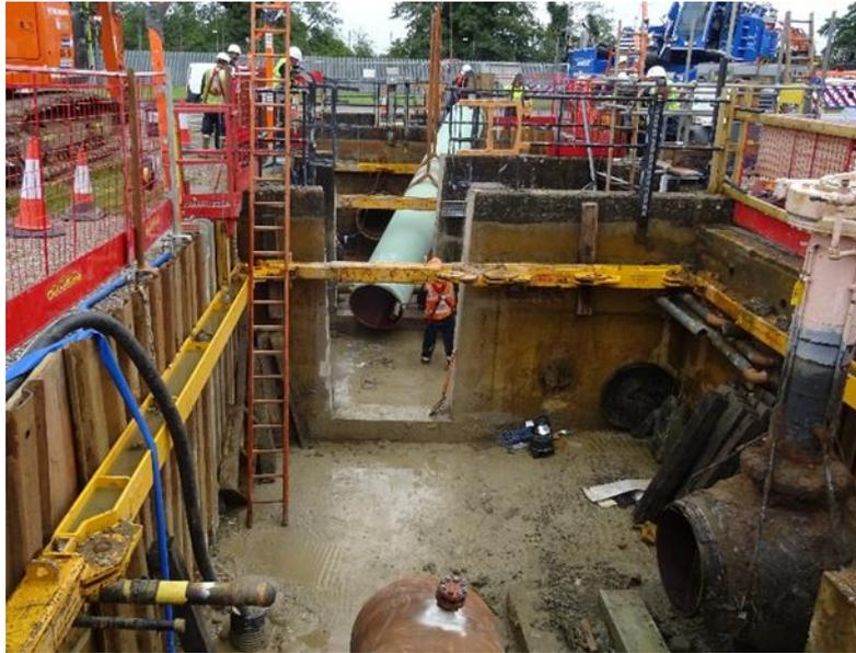
**Figure 17: Deep excavation, valves removed and 36" pipework being carefully manoeuvred beneath the excavation support frames and adjusted into position.**
