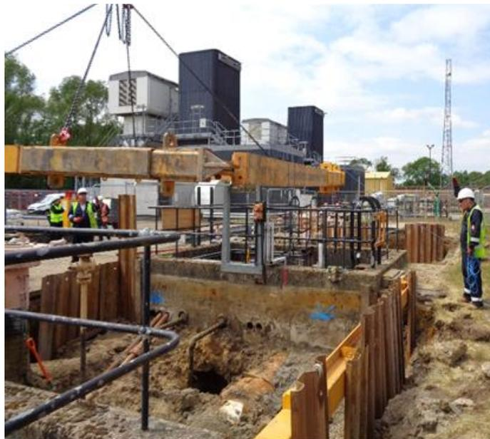
**Figure 16: Excavation with sheet piles and temporary works supporting frame being installed.**
