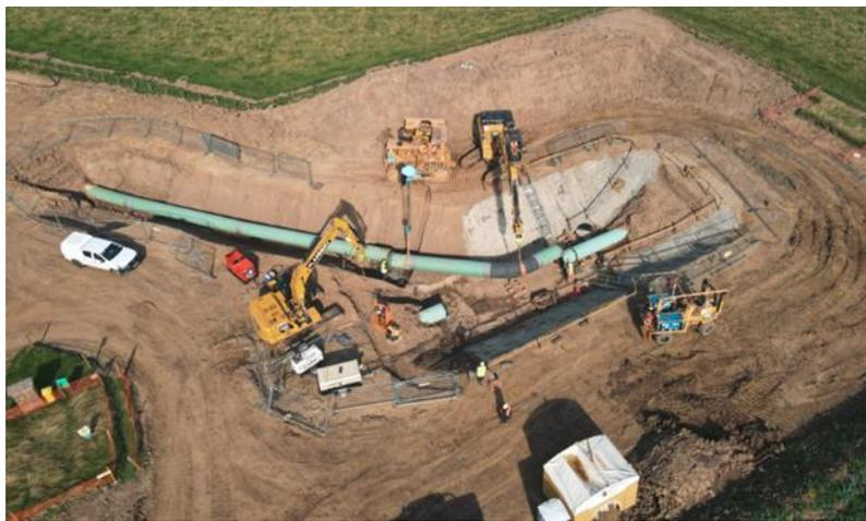
**Figure 28: A1 Morpeth diversion ariel view of tie-in pit final section installation**
