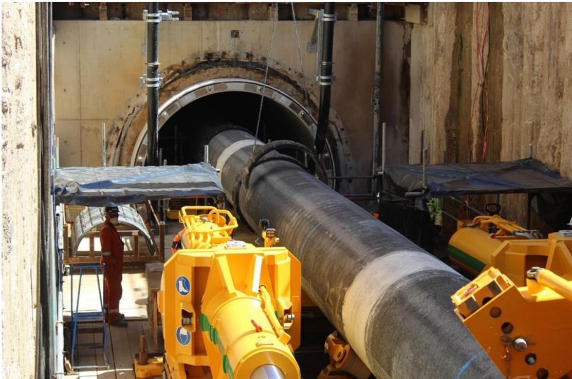
**Figure 20: Pipeline being hydraulic inserted into tunnel – June 2020**
