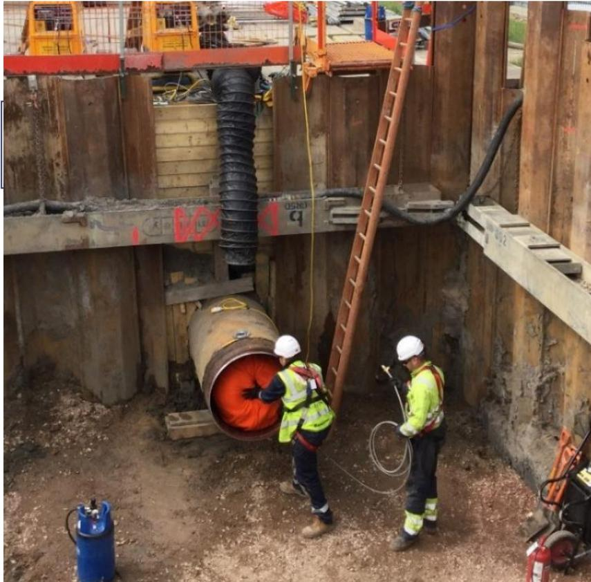
**Figure 25: Bagging process completed at King's Lynn**
