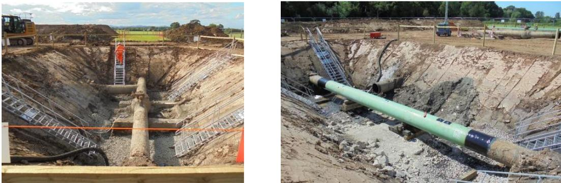
**Figure 20: Excavated Deerhurst West site with previous block valve, and new pipethrough**
