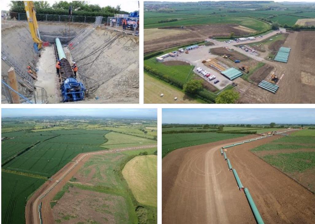
**Figure 37: TX01 Diagrams. (a) Auger Bore Set up at road crossing; (b) Site Establishment; (c) and (d) – Ariel view of pipeline routing following top soil strip and pipe string activities**
