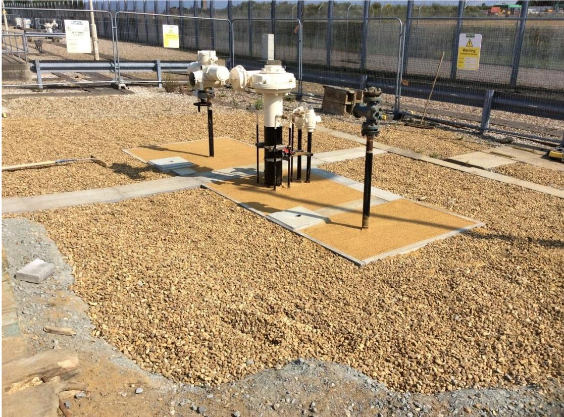
**Figure 8: Installation of Valve FM4/4 approaching installation completion**
