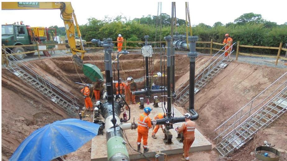
**Figure 17: Installation of Dymock pipework arrangement**
