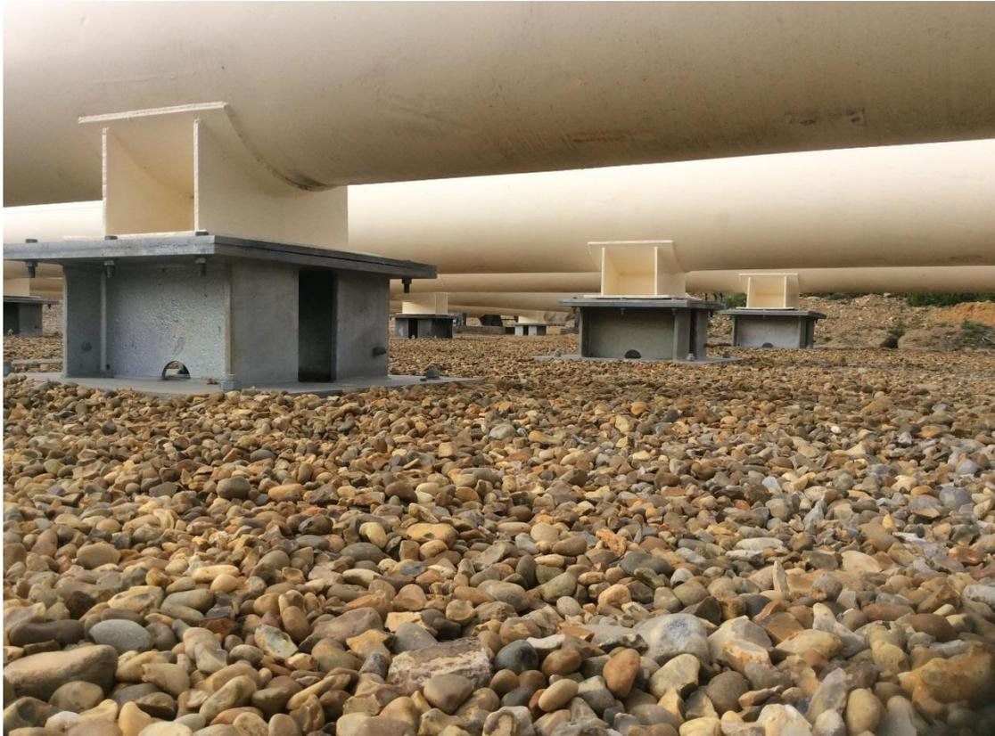
**Figure 10: New-style steel pipe supports installed in Feeder 5 area of site**
