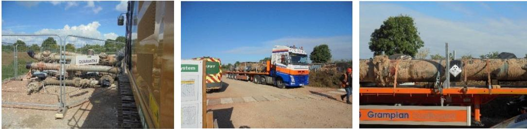
**Figure 23: NORM contaminated waste pipework quarantined and removed from site.**
