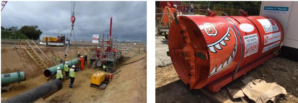
**Figure 39: Diversion works completed via micro-tunnel**
