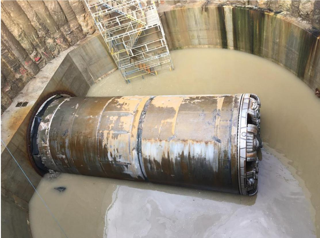
**Figure 28: TBM in reception shaft at Paull (September 2019)**
