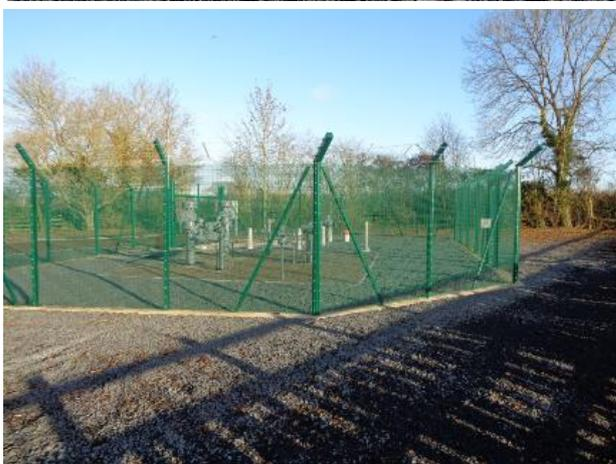
**Figure 18: The completed rebuild of Dymock site, Pipework above ground, ECO Road way, and new security fencing.**
