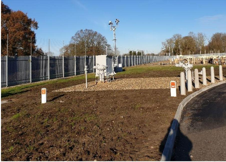
**Figure 26: Completed King's Lynn valve works including new test posts**
