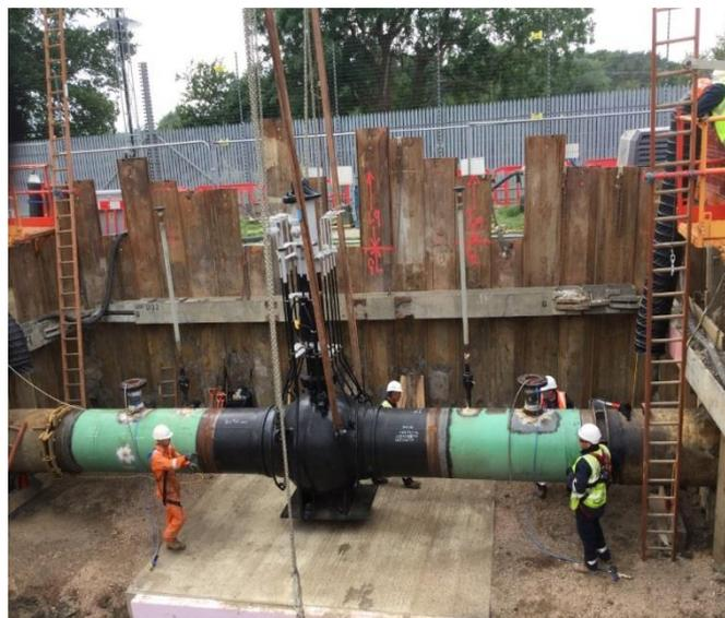
**Figure 24: New valve installation at King's Lynn onto piled concrete foundation**
