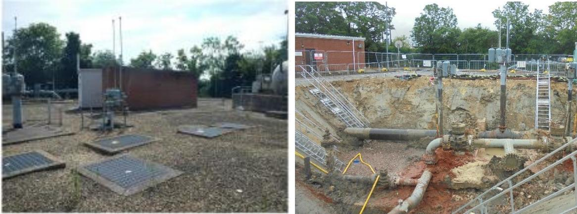
**Figure 14: Photos of Fiddington site valve pits and excavated pipework**
