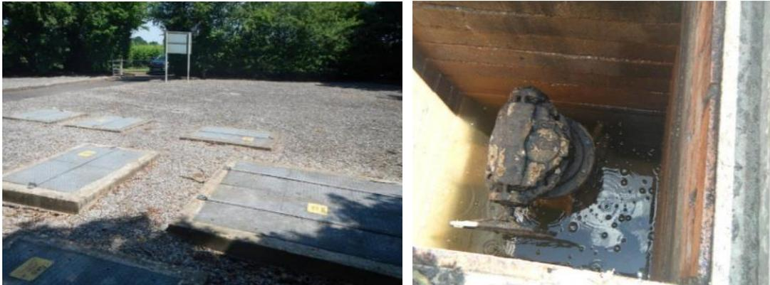
**Figure 16: Dymock AGI with deep pits exhibiting gas leaks**
