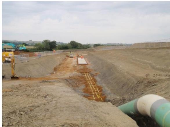
**Figure 38: TX02 Diagram, Deep dig excavation, post pipeline installation and showing the protection slab and marker tape being installed prior to backfill**
