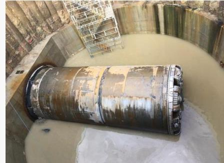
'Mary' our Tunnel Boring Machine (TBM), completes her 5km journey from Goxhill on the south side of the River Humber to the specially constructed shaft at Paull on the north bank.
