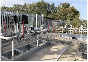
The picture above shows the meter skid (foreground) and filter skid (background) enhancements installed at Eakring
